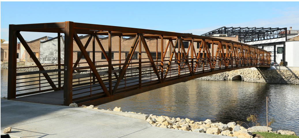
Example of prefabricated steel pedestrian-bicycle bridge.
